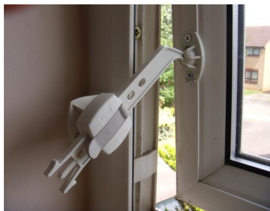
Window Restrictor (to reduce risk of falls)
