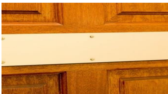
Blanking plate & external letter box
