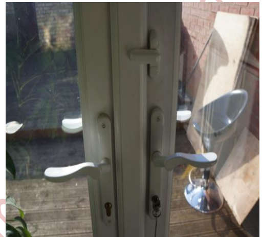
Sash Jammer (fitted to windows & UPVC doors offering resistance to deter forced entry)
