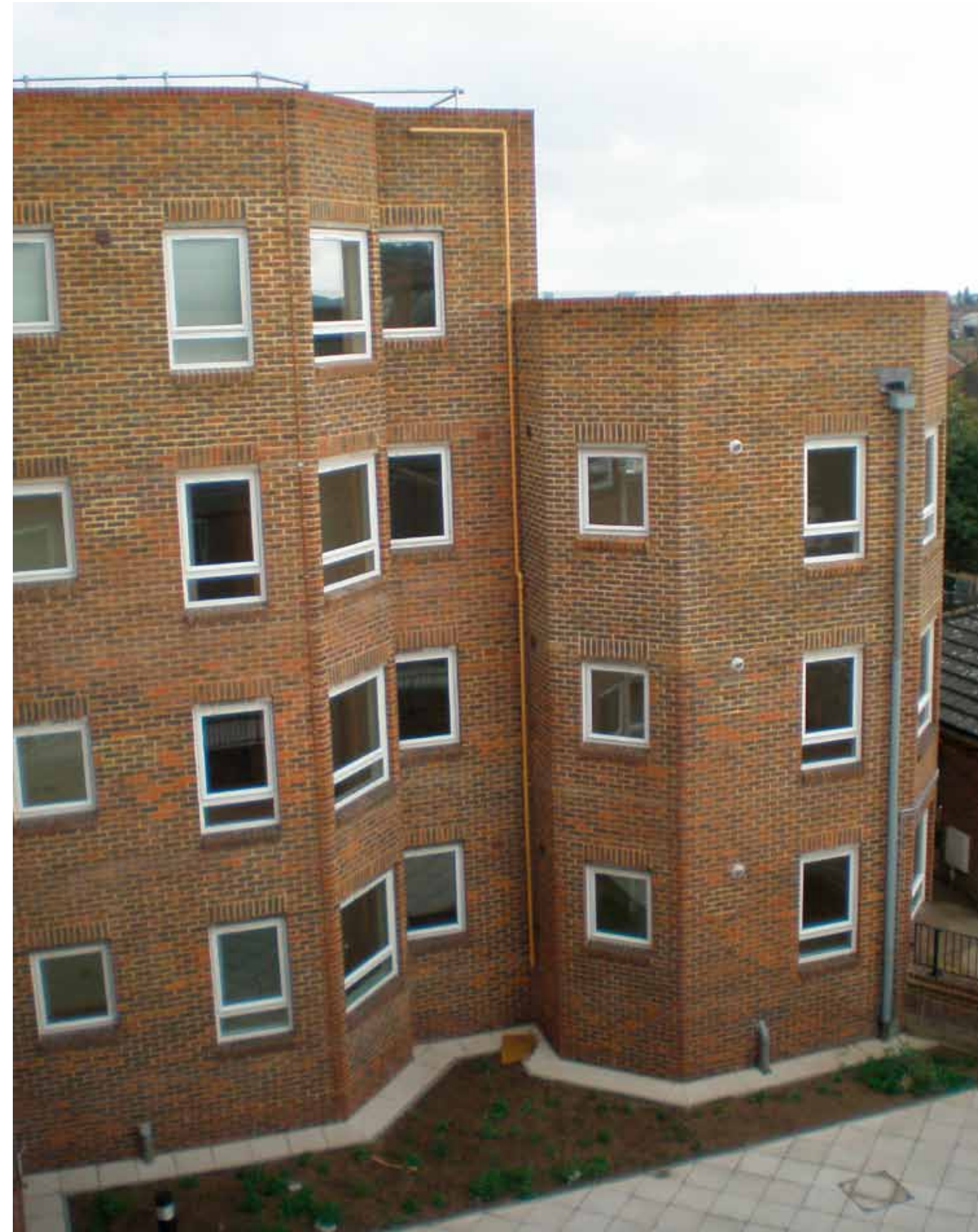
Additional 3rd & 2nd floor extension
