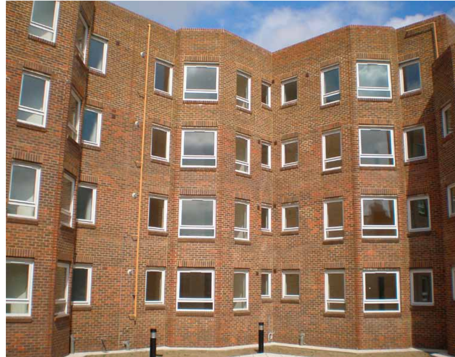
Additional storey added
